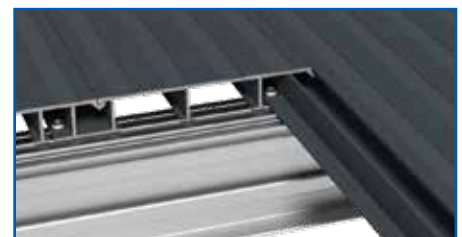
Screw down boards to subframe.
